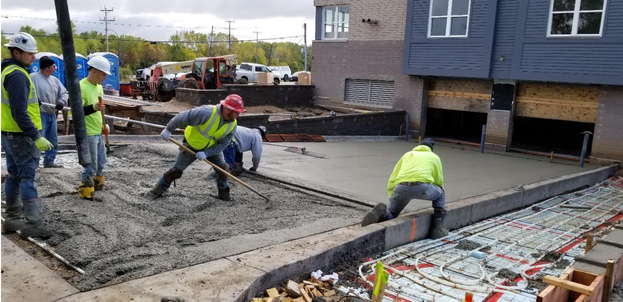
Pouring of drive to underground garage and radiant heat sidewalk
