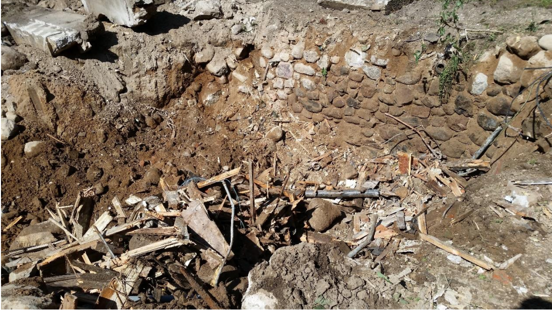
Original Stone Basement Wall
